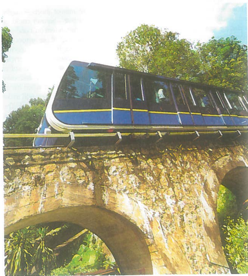
The hill train passing through a bridge.
